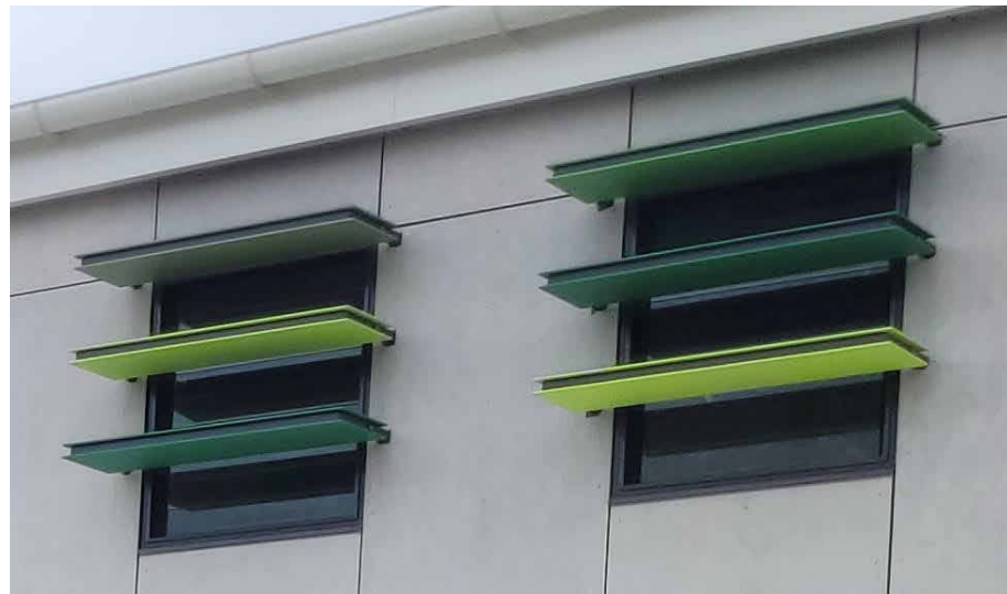
SCD2 Fixed horizontal sunshade blades in feature colours
