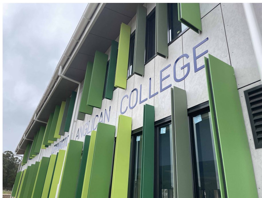
SCD1 & SCD3 Fixed vertical sunshade blades in feature colours
